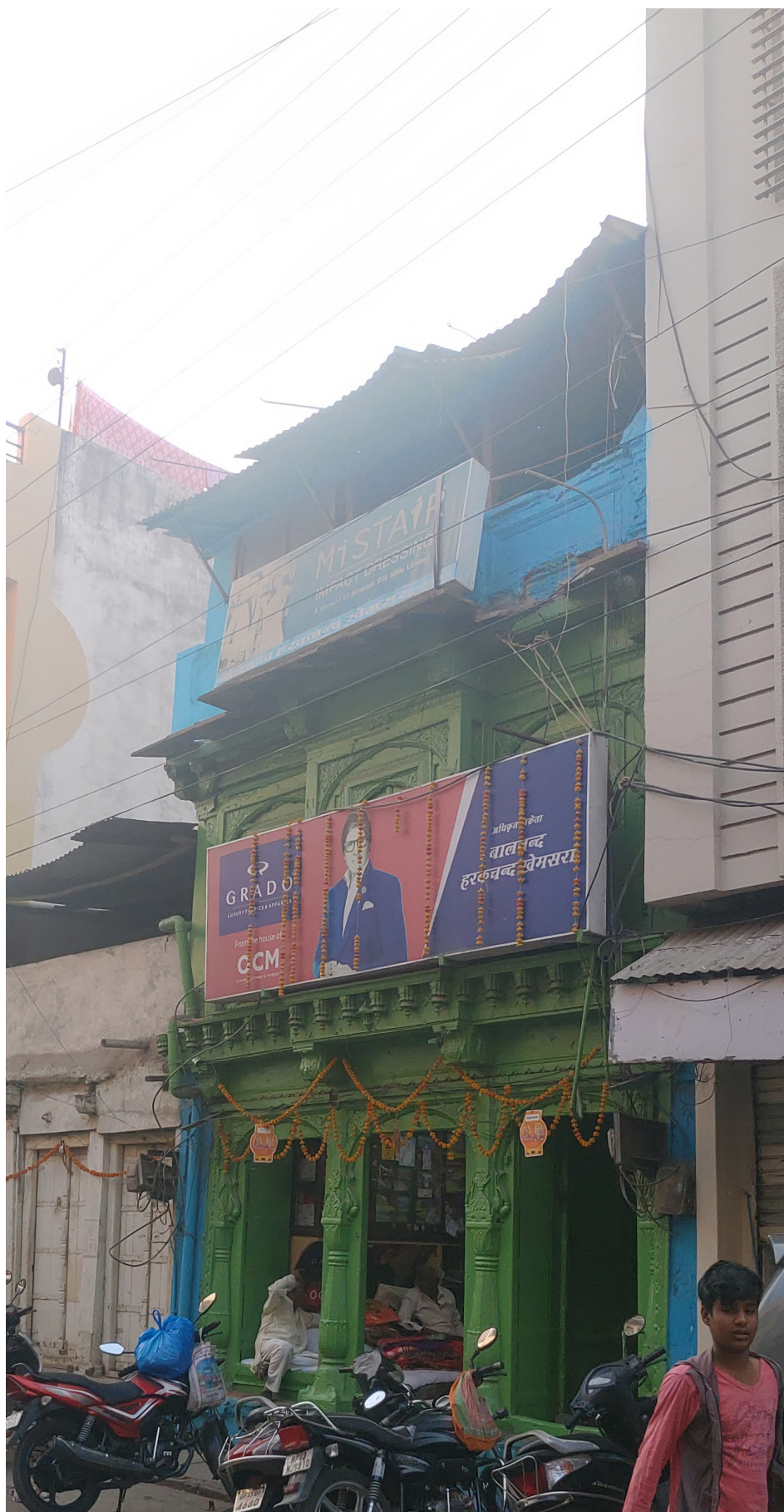
Figure 42 : Insensitive additions and alterations on a heritage facade, Hatta.
