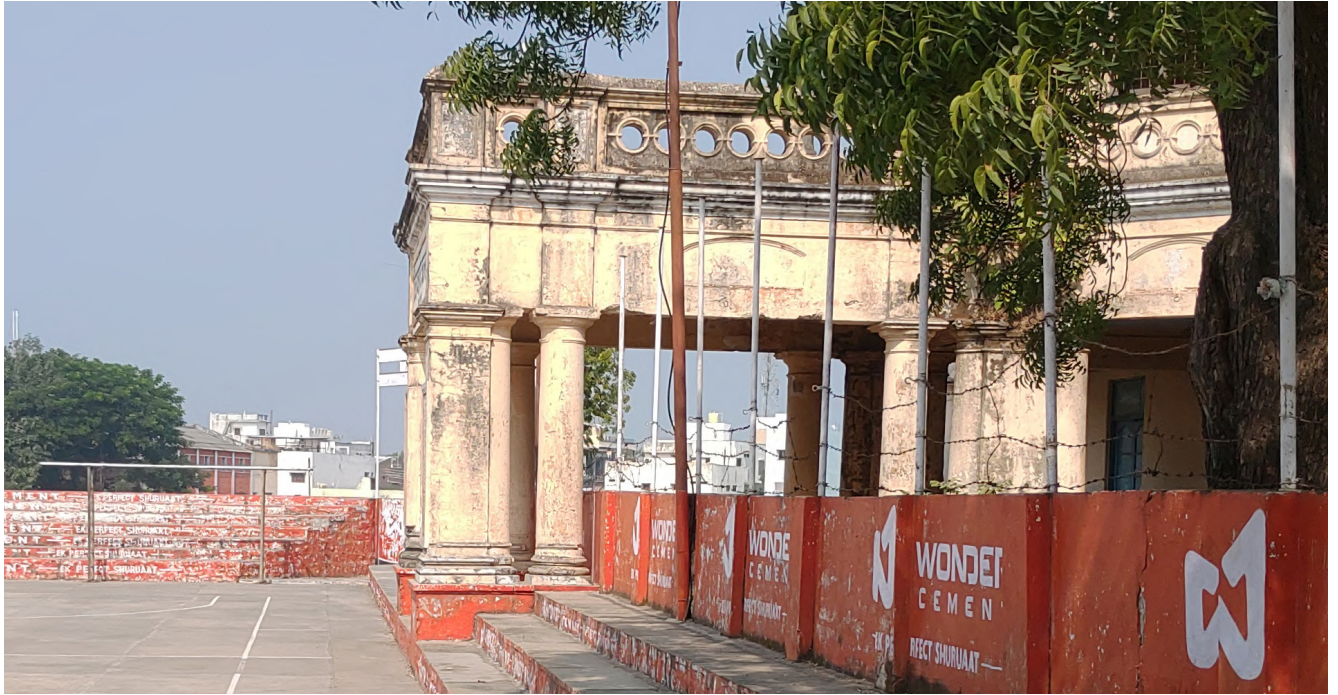
Figure 40 : Disregarded development around porch of a palace at Jaora
