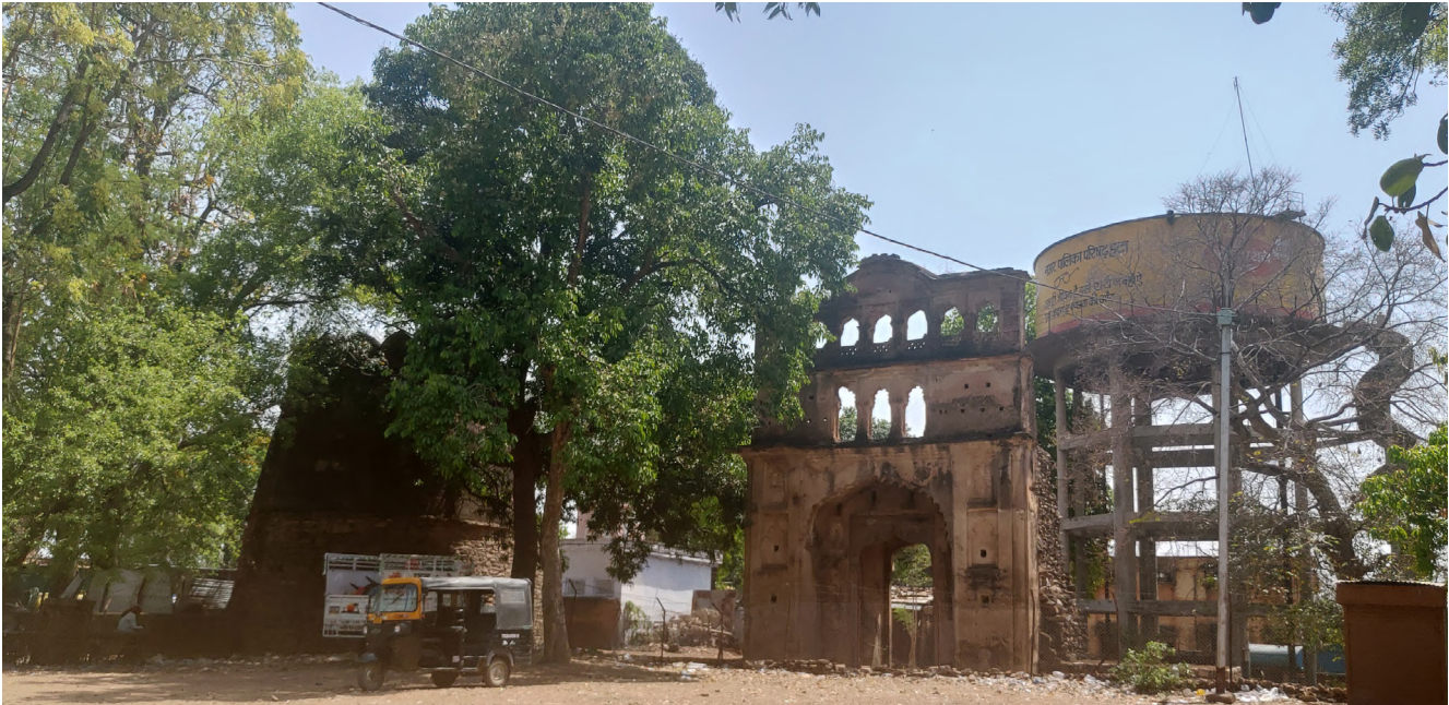
Figure 44 : New structures supressing tangible heritage at entrance gate Hatta fort
